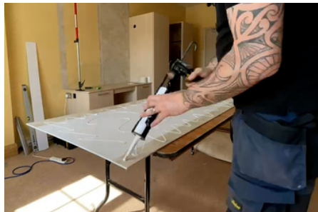
STEP 2 - GLUE THE FOAMALITE® SHEET
